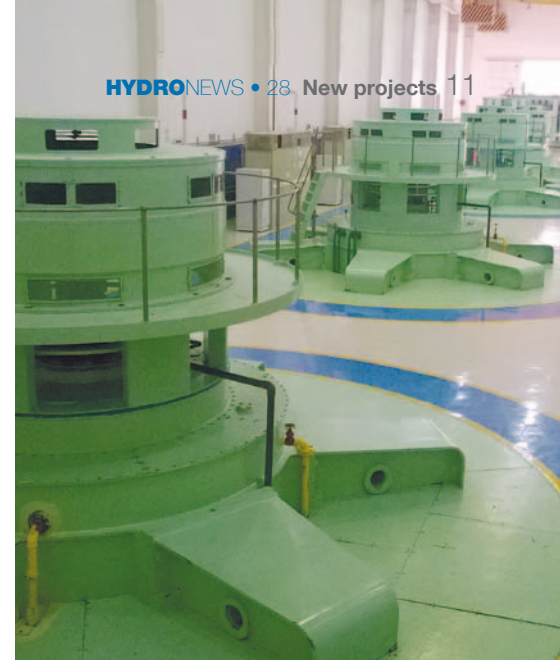
▲ Units #1 – #4 before rehabilitation
