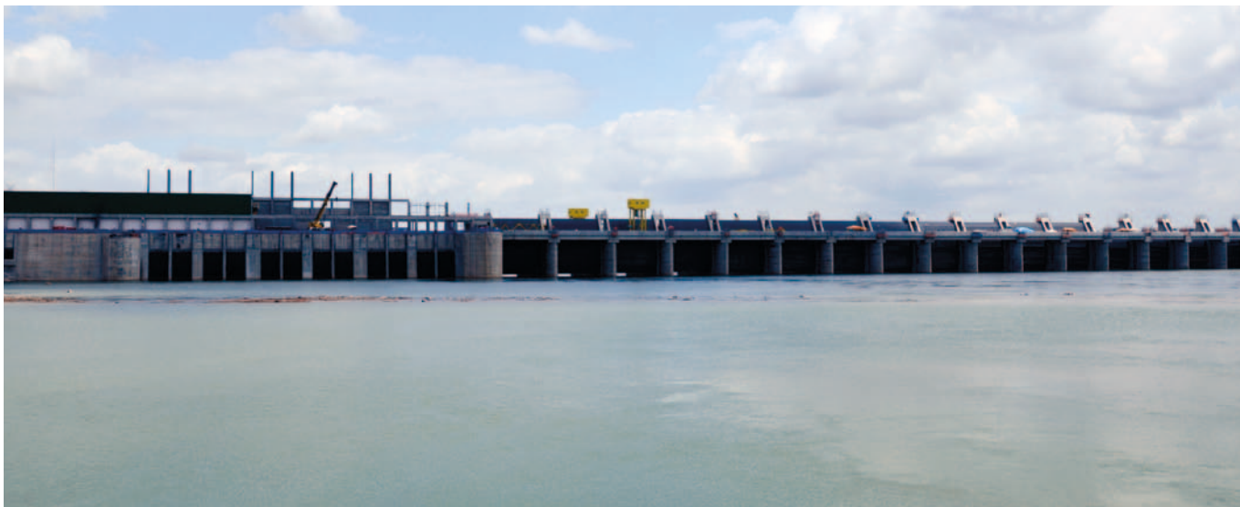
▲ Belo Monte spillway at Pimental site
