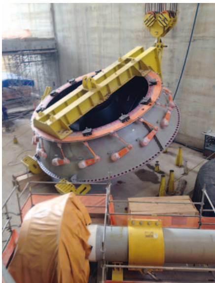
▼ Installation of distributor at HPP Pimental
