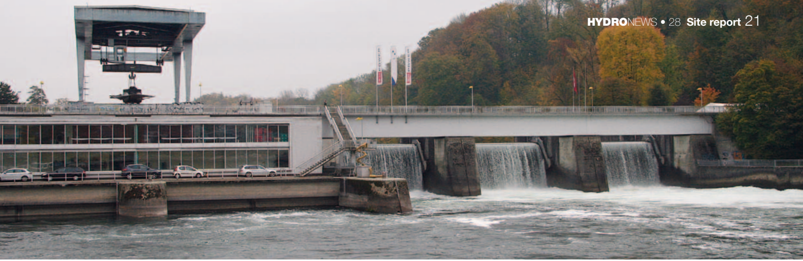
▲ Hydropower plant on the Rhine River
