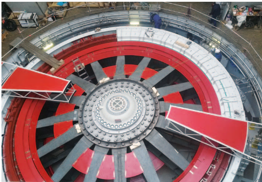
▲ Installation of covers and air shield
