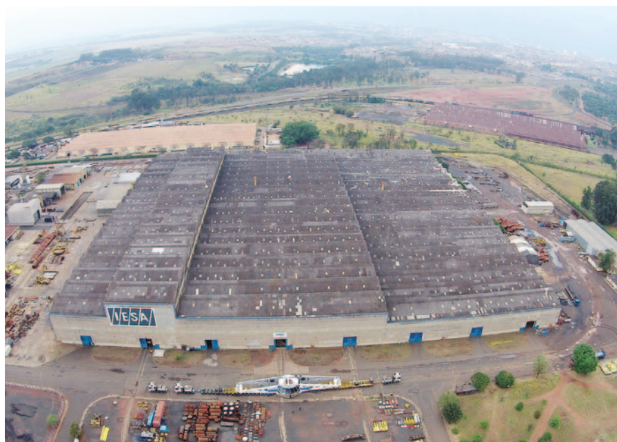
▲ IESA plant in Araraquara and runner of HPP Belo Monte during transport
