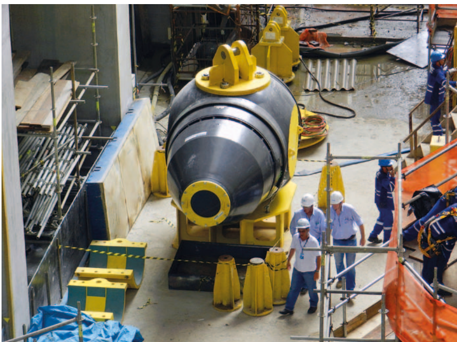
▼ Kaplan runner installation at HPP Pimental
