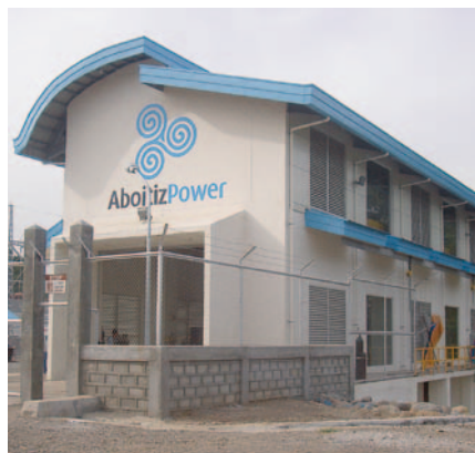
▼ Powerhouse of HPP Tudaya 2
