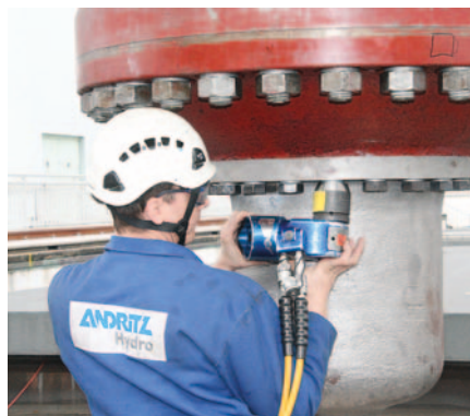
▲ Preparations for reassembly
