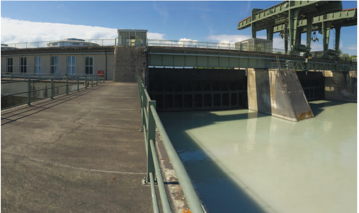
▲ Rosenheim hydropower plant
