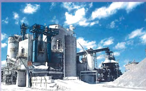
Western Lime Corp.'s Green Bay plant.
