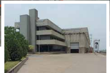
▲ Kpong hydropower plant
