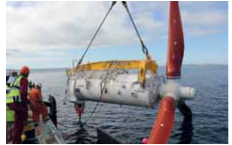
▲ Installation at EMEC site
