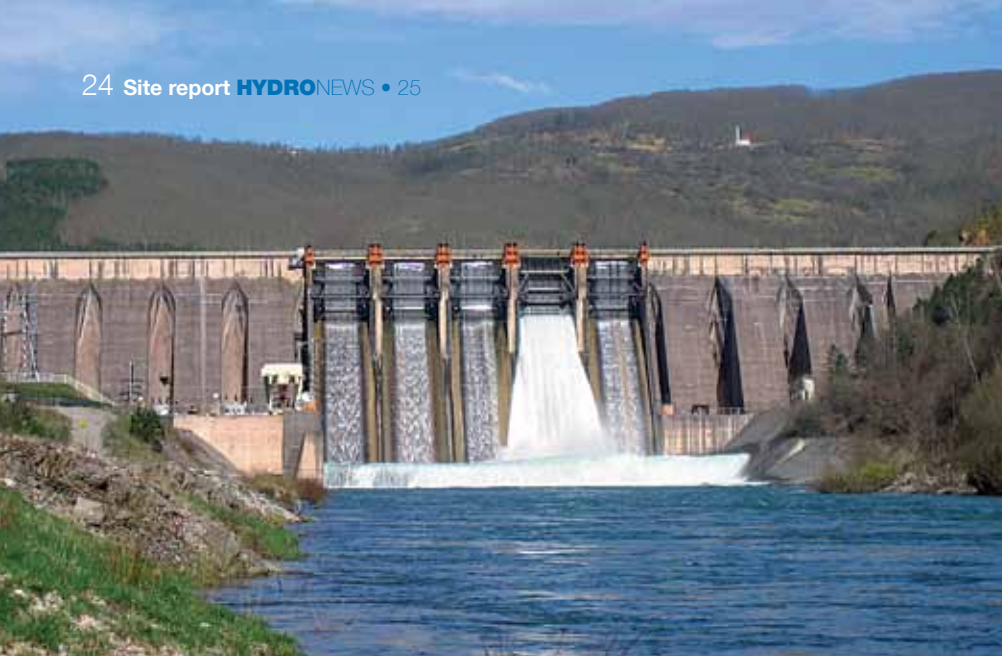
▲ View of Bajina Bašta hydropower station
