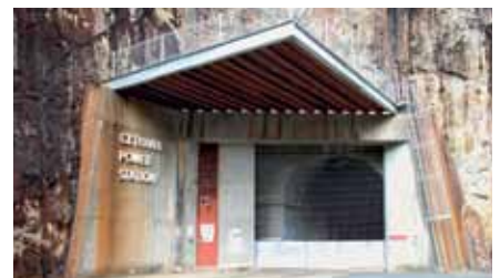
▲ Entrance to the power station tunnel at HPP Cethana
