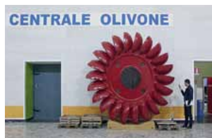
▲ Centrale to be replaced by Powerplant
