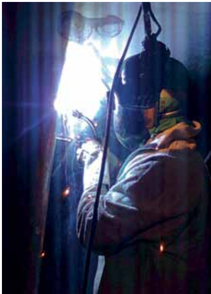
▲ Cavitation service repair in HPP Taquaruçu
